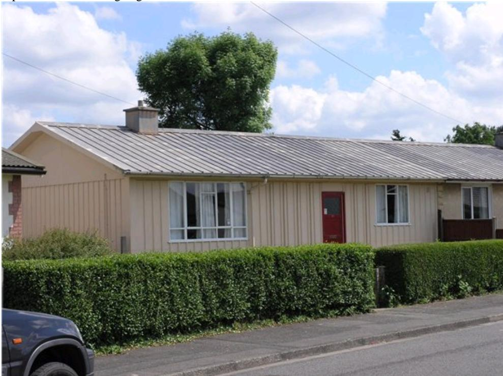
**Figure 2 Bungalows have steel panel construction with panels or render on the façades. Many retain their original walls and roofs, although almost all have replacement doors and windows**
